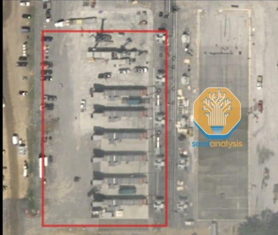
xAI Colossus 2 - seven Titan 350 turbines (266 MW) Source: SemiAnalysis Datacenter Industry Model
