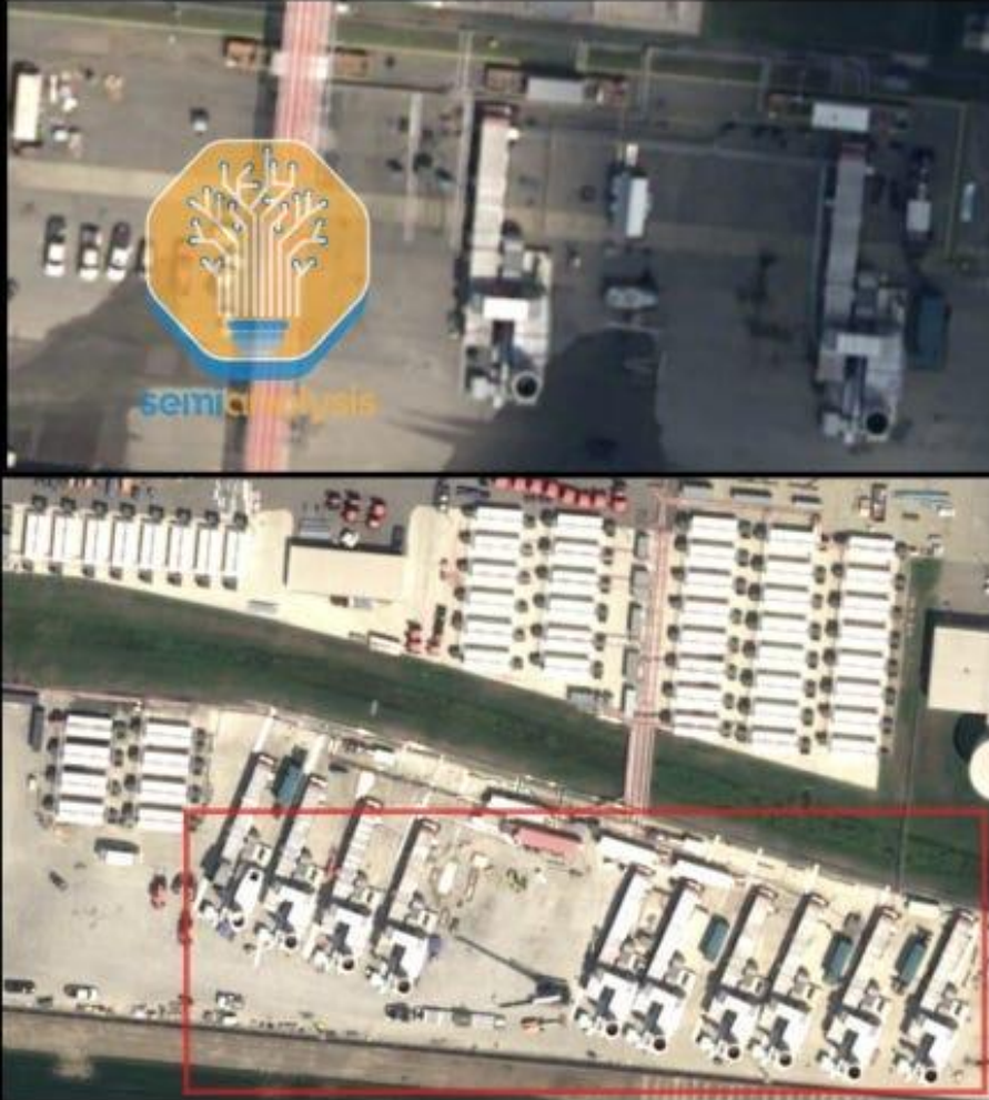
xAI Colossus 1 - twelve SMT-130 turbines (198MW) Source: SemiAnalysis Datacenter Industry Model
